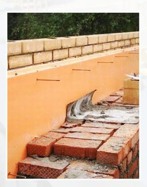
Flexible bonds of polymer composites are used to interconnect layers within outer multilayer walls. This technology is often used to construct buildings with improved thermal insulation properties.
